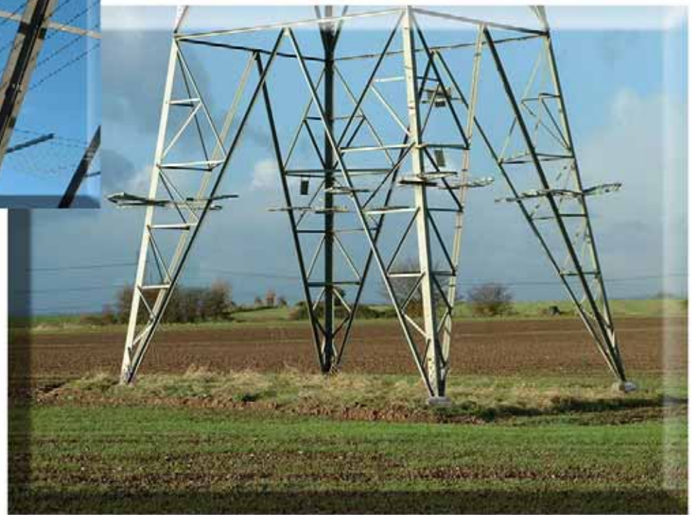
275kV AND 400kV NGC TOWER ACD's
